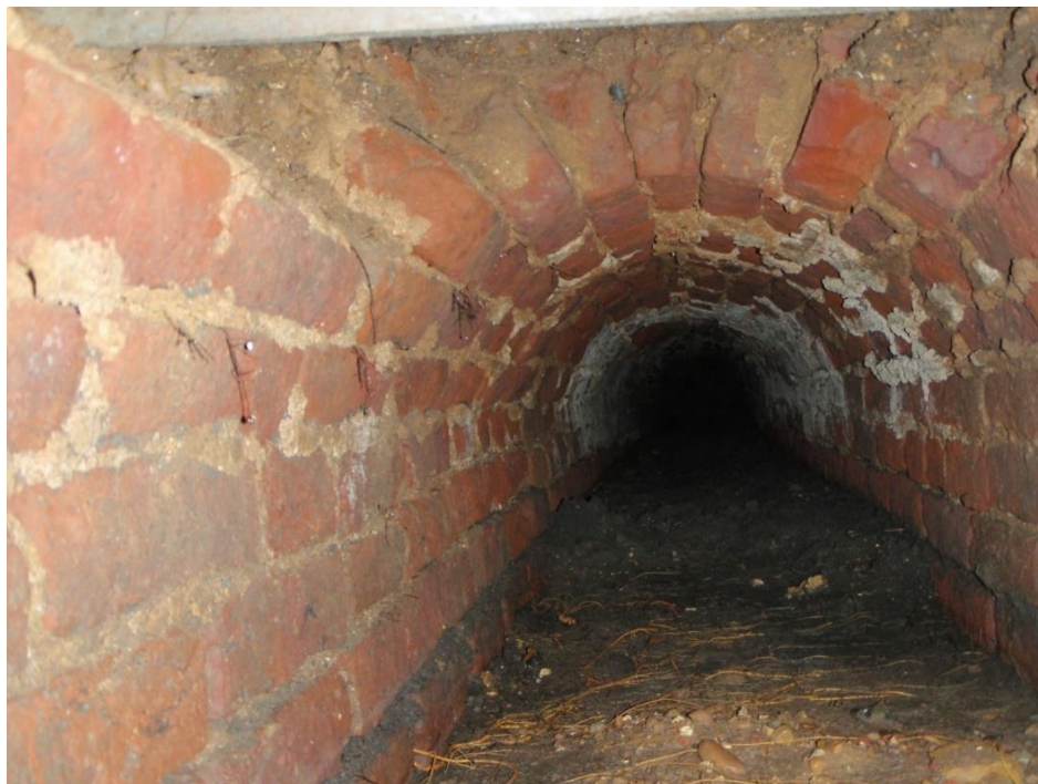
Pl. 46: FXA10 D1; Internal View South West Along Phase 2/3 Drain [10212]
