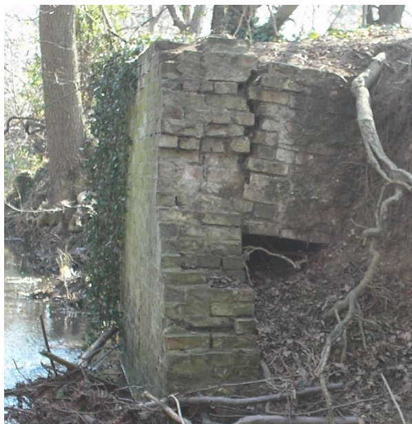
Pl. 70: The 'Tie Back Wall Behind the South Retaining Wall
