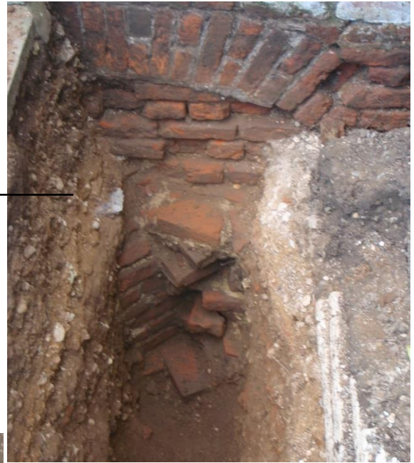
Pl. 16: FHN09 Trench 3, South Elevation of Standing Wall Showing the Phase 3 Relieving Arch and Drain [09113]/[09131]
