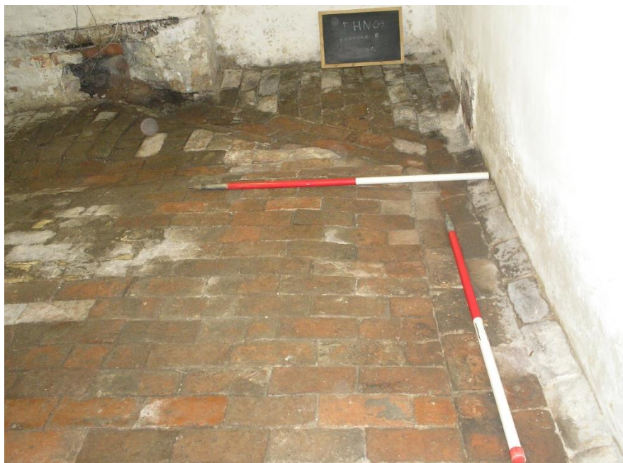
Pl. 22: Extant Brick Floor in Basement Room A006 Showing the Gutters Running into the Phase 4 Lead Channel Through the West Wall
