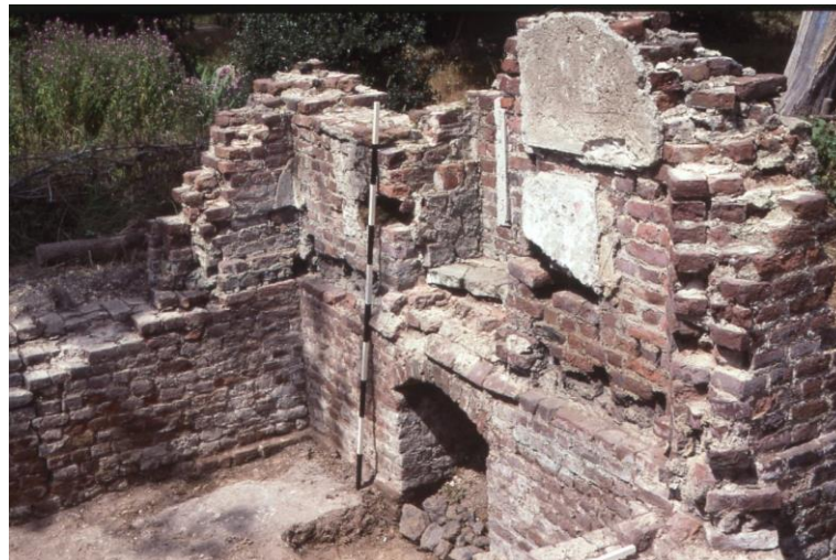
Pl. 58: The Interior of the East Summerhouse Looking North, Showing the (Sub)Basement Arched Support to the Partly Lost Fireplace Above (photo Geoffrey Gillam (© Enfield Local Studies Library))
